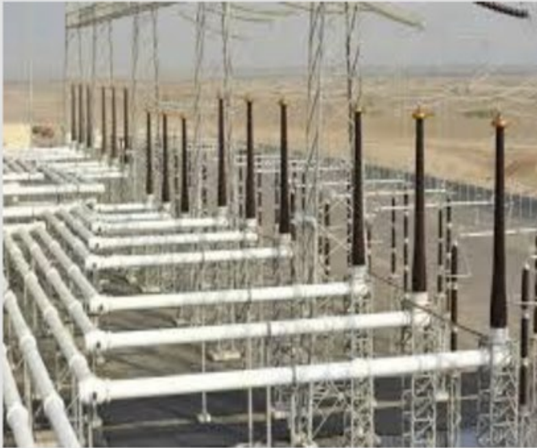
AREVA T & D - Dubai, UAE Modification works on 11kV GIS switchgear, install & wire, CTS Energy meter, test plugs etc in
