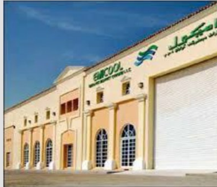
Emicool Dubai Investment Park Rectification containment blockage for communication Fiber Optic Cable - Dubai
