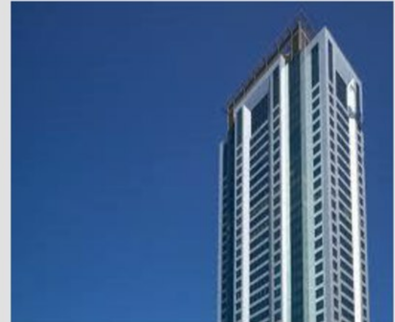
Al Hatboro Specon Cable Glanding & Termination Works for HS103 Jumeirah Beach Residence - Hotel at Dubai
