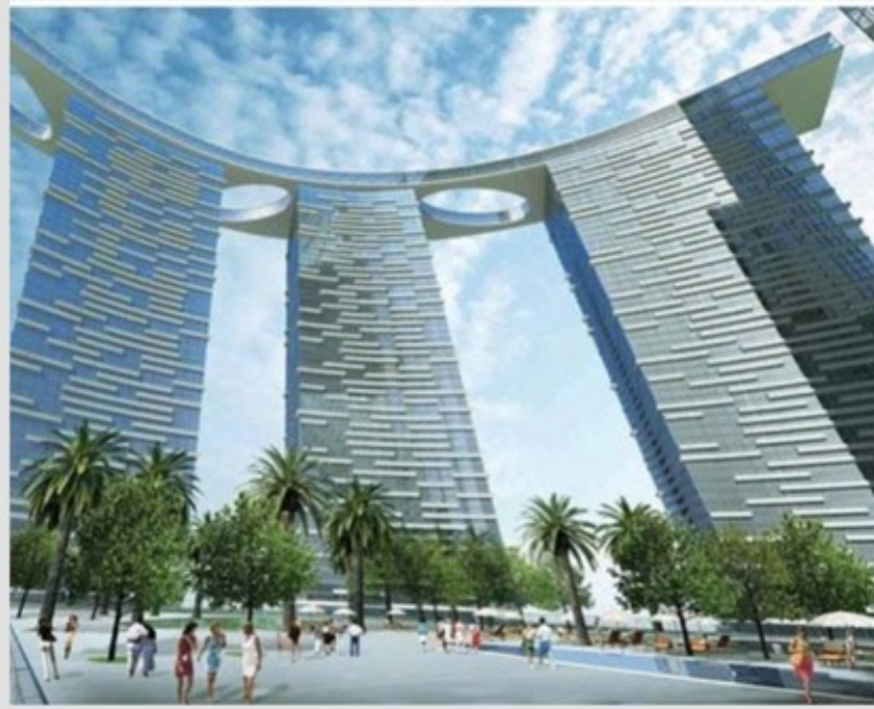
Project Name: Sun and Gate Distracted Tower Location: Al-Reem Island, Abu Dhabi Description : G-I Duct installation with Thermal Insulation & accessories
