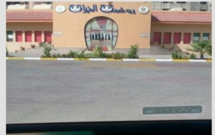
Al Hayat Kindergarten We are also still working on this school) MEP Works
